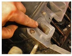
I smeared a thin layer of RTV silicone (which came with the new intake gaskets) over the pitted areas around the cooling passageways.
