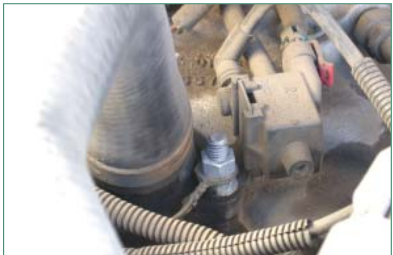
Figure 4: DRAC ground (G134) on thermostat housing bolt
